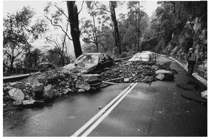
Figure 3.1a Road damage following flooding/landslides Illawarra, 1998
