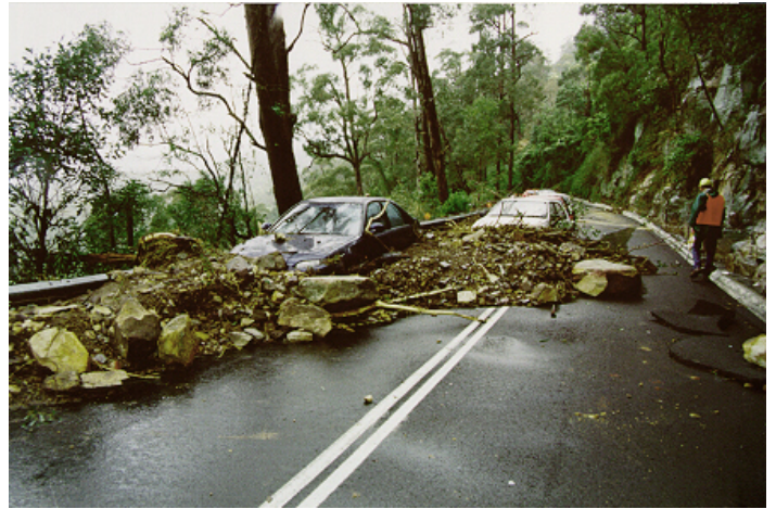
Figure 3.1a Road damage following flooding/landslides Illawarra, 1998
